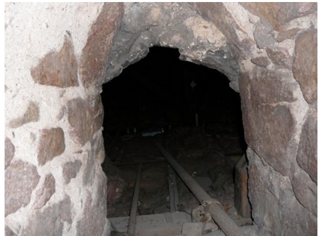
St Peter’s – tower opening into the body of the church
