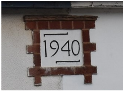
11 Near Hawthorn Road
