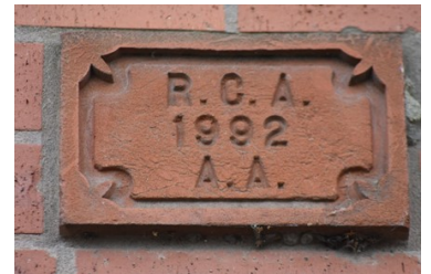
3 On Loughborough Road near Bond Lane
