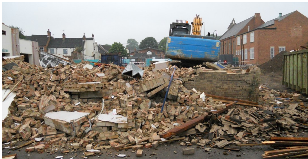
25 th August 2016 Demolition underway
