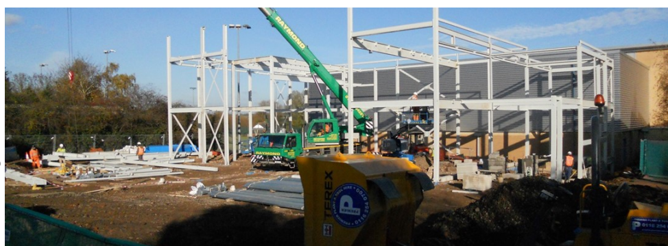
11th November 2016 Construction of the new Centre underway
