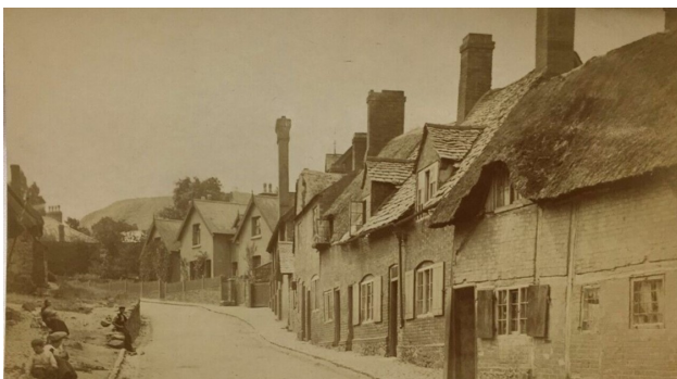
Watling St looking west c1880 following the construction of St Peter's School
