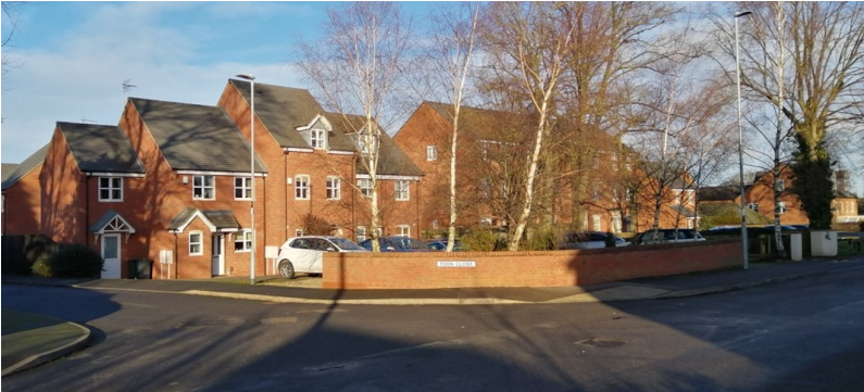
The site of The Lindens December 2020
