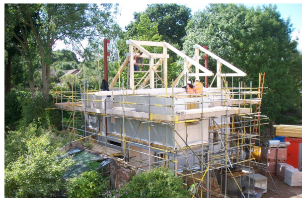
Building the Eco House
