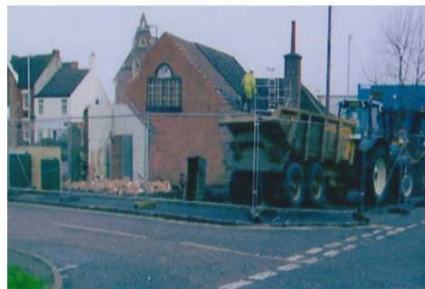
Renovation in progress
