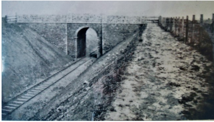
Deep cutting at Bond Lane
