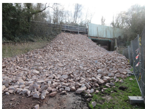
Before the repairs started
