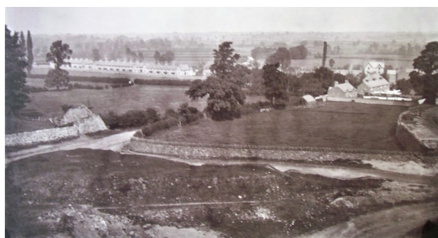
Bond Lane before the bridges were built
