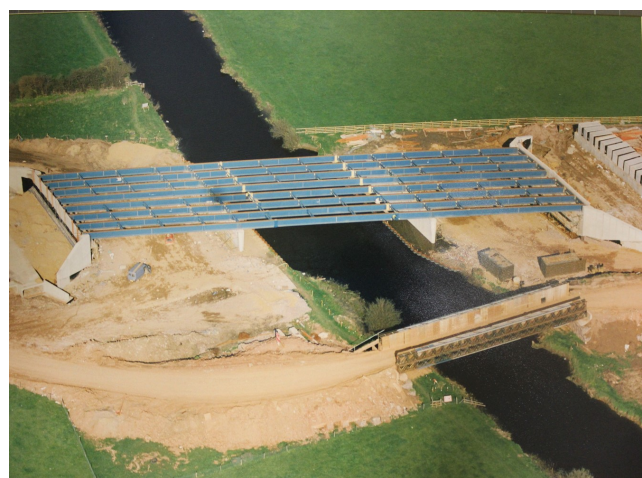
River Soar Bridge No 3 being built to take the bypass
