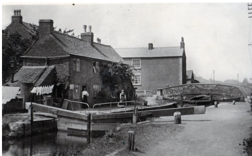
Lock Bridge No 24, a typical brick hump backed canal bridge. Written on the back of this card
