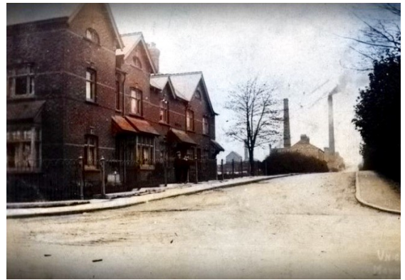
Brickyard chimneys at the top of Union Lane
