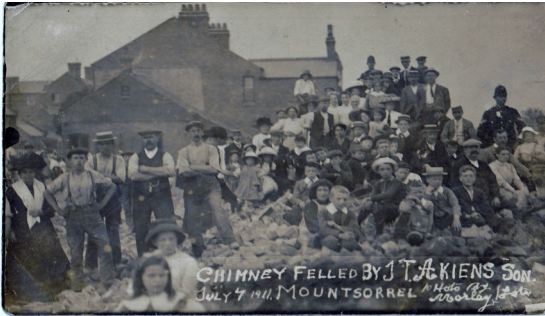
Demolished chimneys somewhere in Mountsorrel
